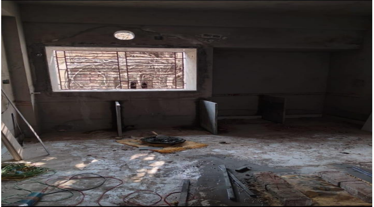
1A kitchen counter work going on.
