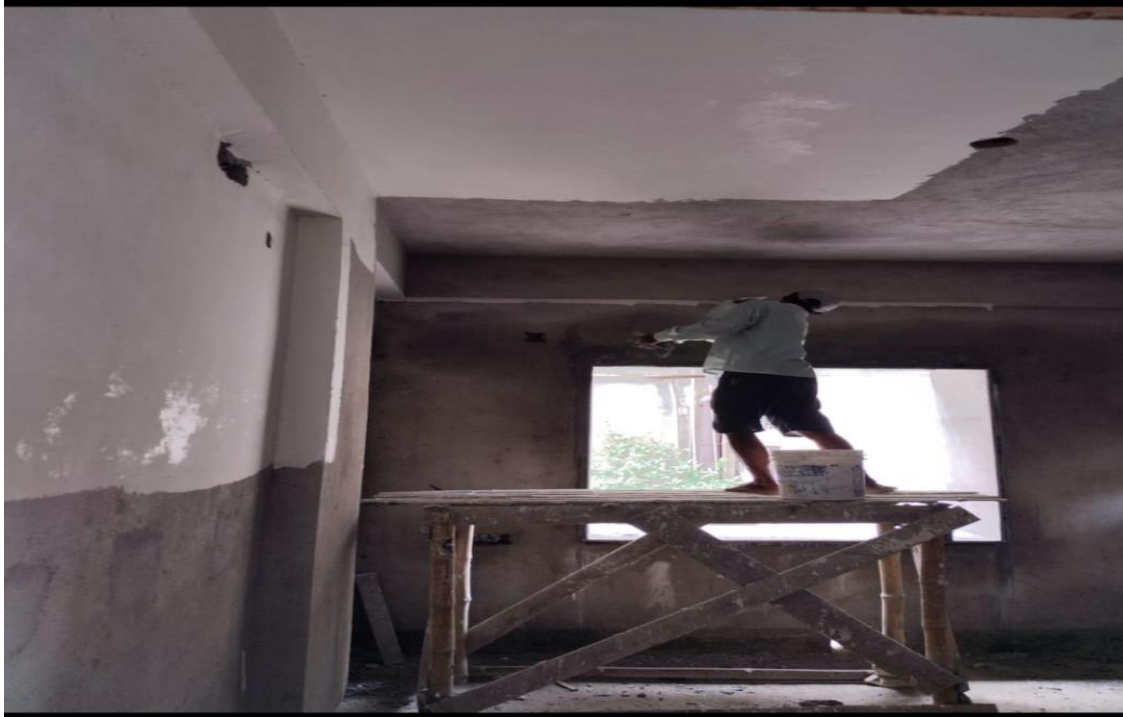
Putty work inside flat started
