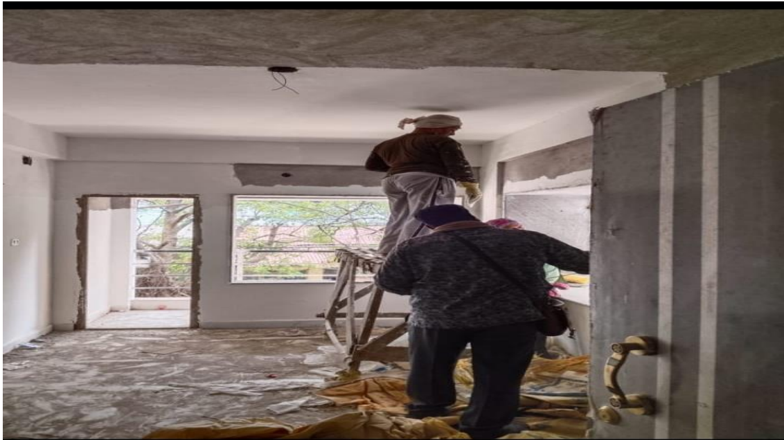
1D putty work going on
